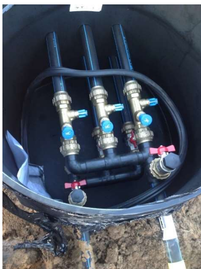
Manifold chamber from above
