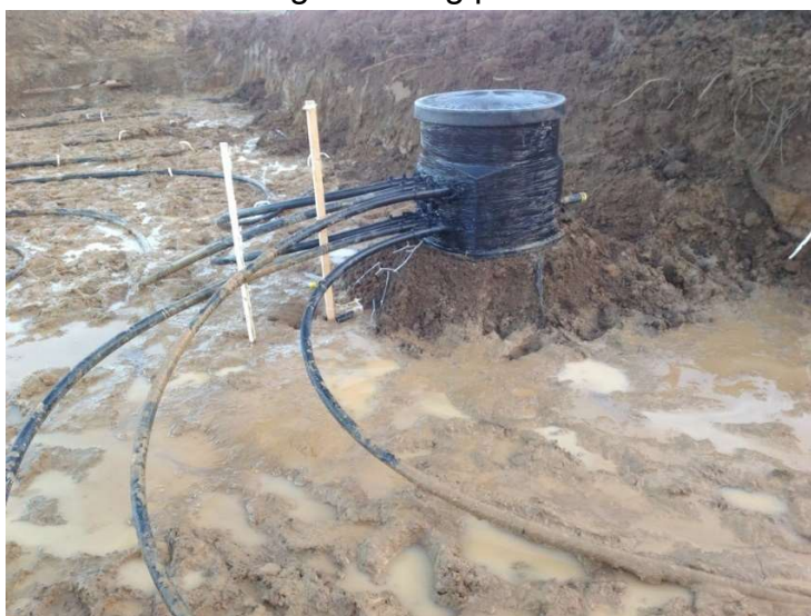
Manifold chamber with lid prior to back-filling
