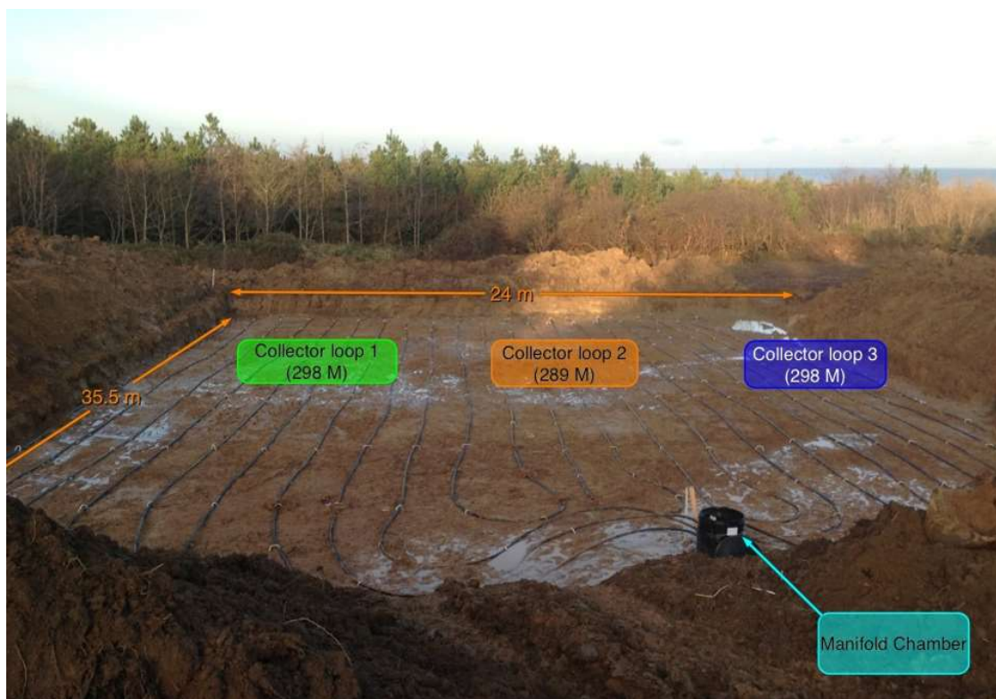
Three-loop collector field for a large house – no pipe joints in the field, only inside the manifold chamber
