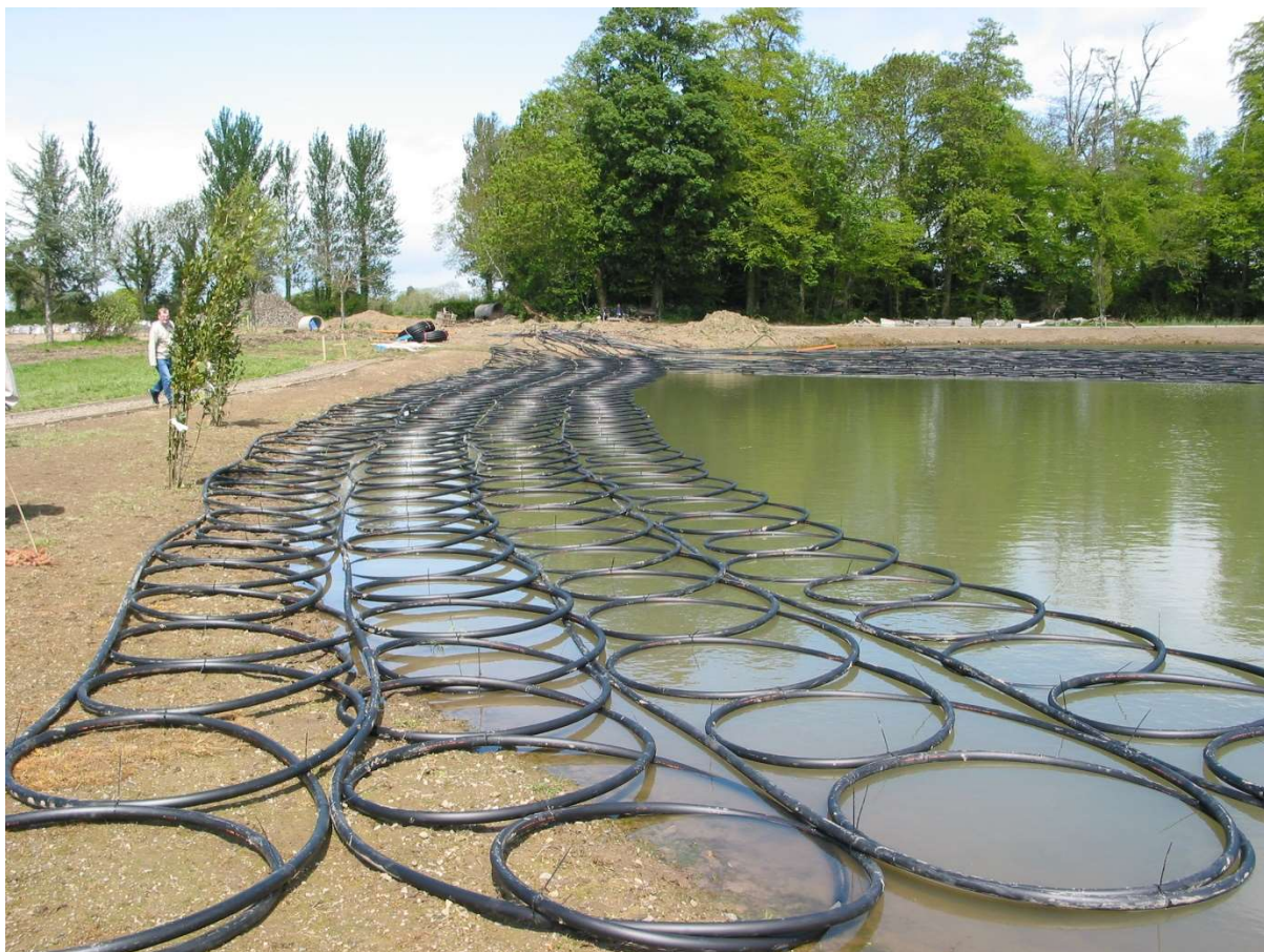
Collector on the shore before sinking with weights to the lake bed for a large Irish period country house. The 5-acre lake supplies the sole source of heat for the 26,000sq. ft. house plus a swimming pool.
