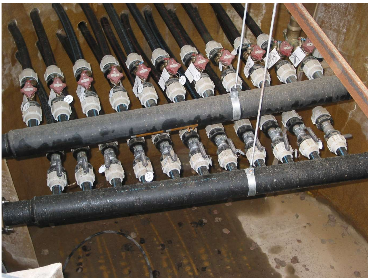
Manifold chamber for a large lake collector with valves and flow regulators.
