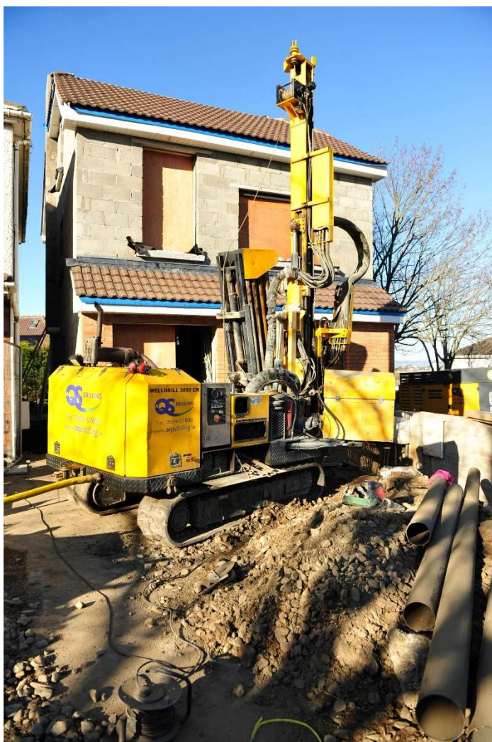
Mini Drilling rig making a borehole in a suburban Dublin house- with a tiny garden, the owner elected to use a borehole as the more aesthetic solution over an air to water heat pump.
